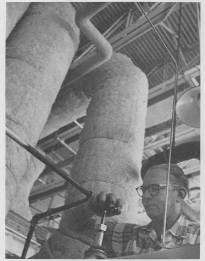
AIR CONDITIONING installation for the 705 EDPM facility is extensive. Vern L. Brockway (2411-2) makes final adjustments on the absorption refrigeration system of the cooling system.
